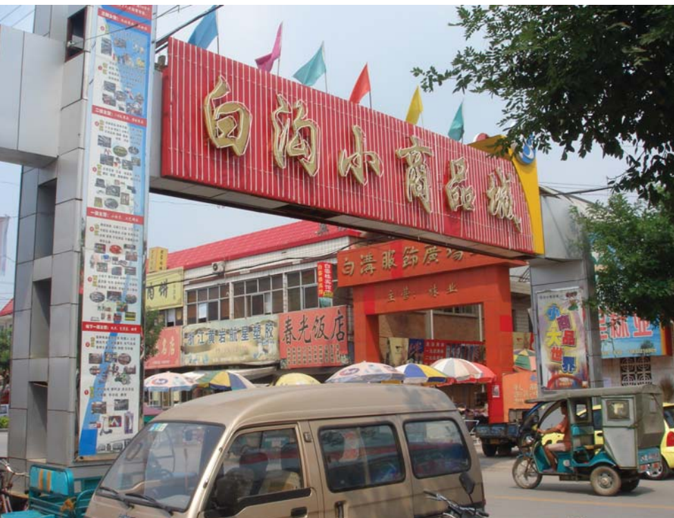
A building specializing in small items faces this street. Sign with information on the small items building. Another sign on the pillar on the left gives information on the products.
